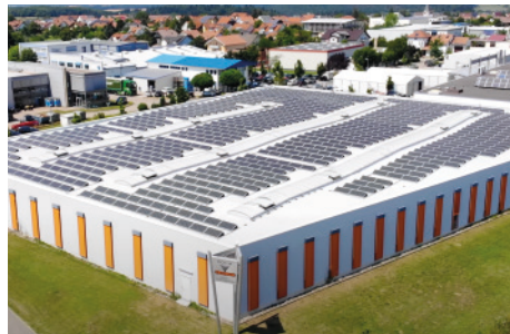
Factory II: Dryer construction facility in Göbrichen
